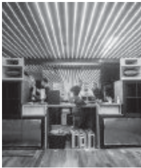
The Phuture Sound team installing the system
